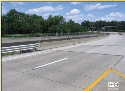
A new rail system will be installed atop the existing bridge barriers providing additional safety for cyclists.
